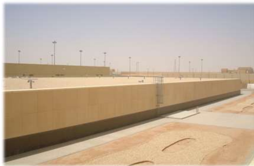
Potable Water Tank
