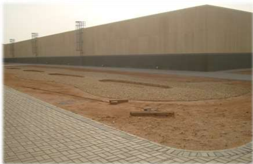
Irrigation Water Tank
